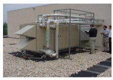
The true desiccant system is actively regenerated, as opposed to passively regenerated by the requirement of cooler, drier exhaust air. The actively regenerated system does not require exhaust air to function; however, energy can be recovered from the hospital's exhaust air if desired and practical. The actively regenerated desiccant system also includes two to three times the amount of desiccant material, as does an enthalpy, or energy recovery, rotor.
