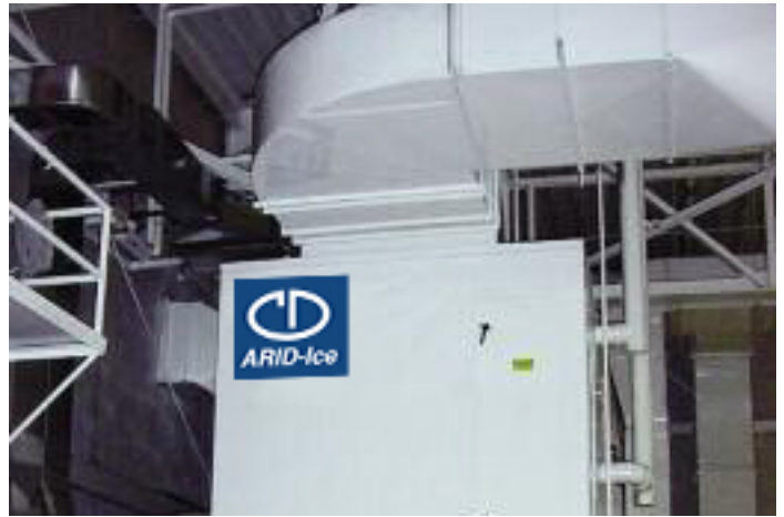
Indoor installation rated at 12,000 SCFM.
