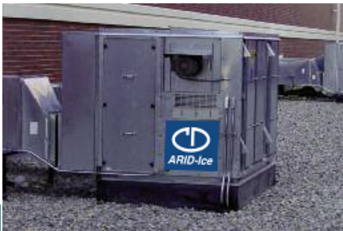
Rooftop installation rated at 5,500 SCFM
