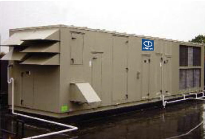
Rooftop installation rated at 10,000 SCFM
