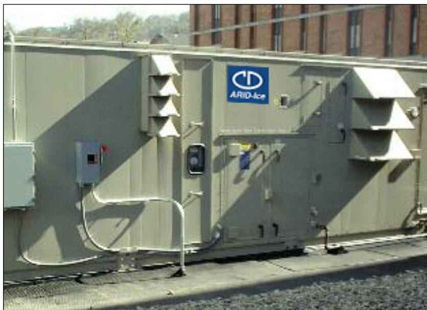
Rooftop installation rated at 15,000 SCFM.
